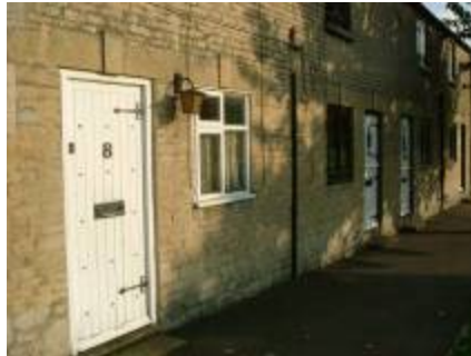
Modern replacements of 19 th c. sash windows, panel doors and 18 th c. plank doors.
