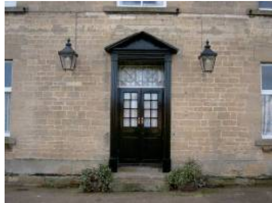
19 th c. door, fanlight and case, slightly modified in the 20 th c.
