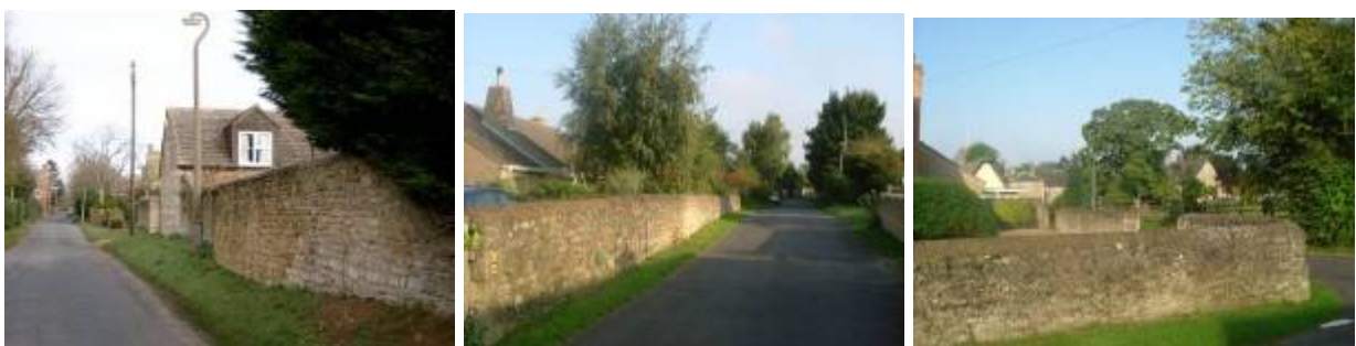
Walls in the townscape
