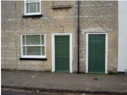
19 th c. doors & windows replaced in replica
