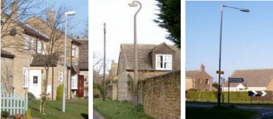
Some of the styles of lamp-post in the conservation area.
