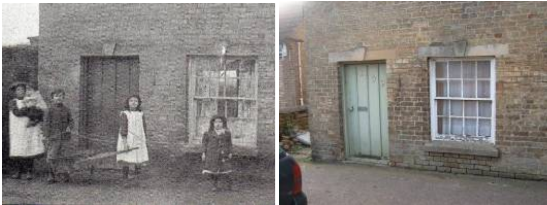
19th c. beaded plank door and sash window - surviving to this day - 105 Peterborough Road
