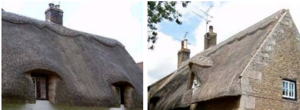
Longstraw thatch roofs with hooded gabled or eyebrow dormers
