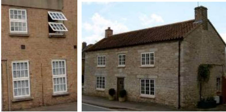
20th c. sash and casement replacement windows.
