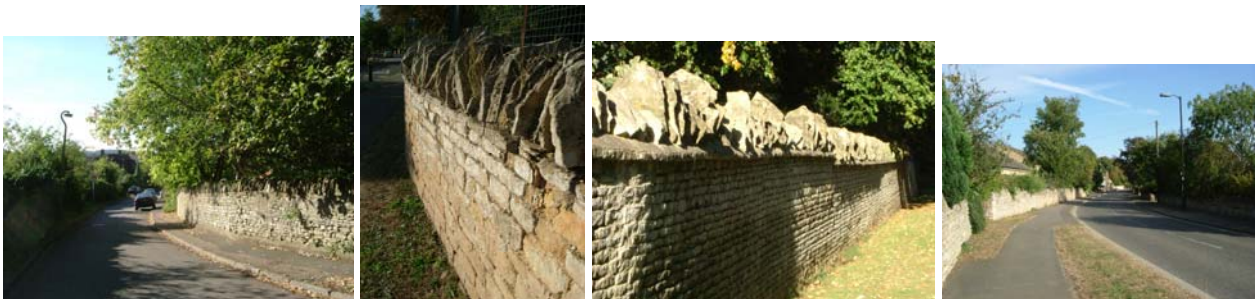
Major presence of stone boundary walls
