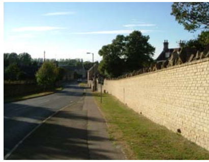
Boundary wall to Castor House
