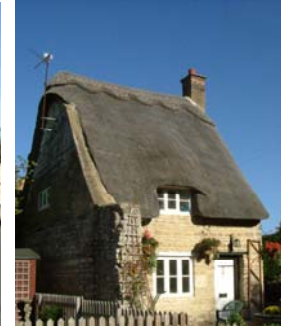
Squared rubble stone and dressed stone quoins, stone lintels (Collweston and slate roofs)
